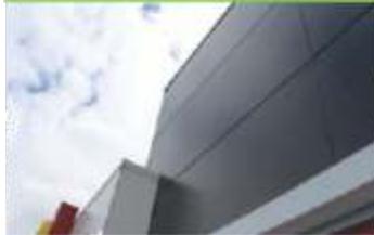
Finishing: Fibre Cement
